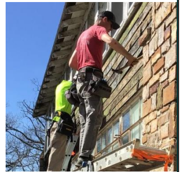
Installing shakes
